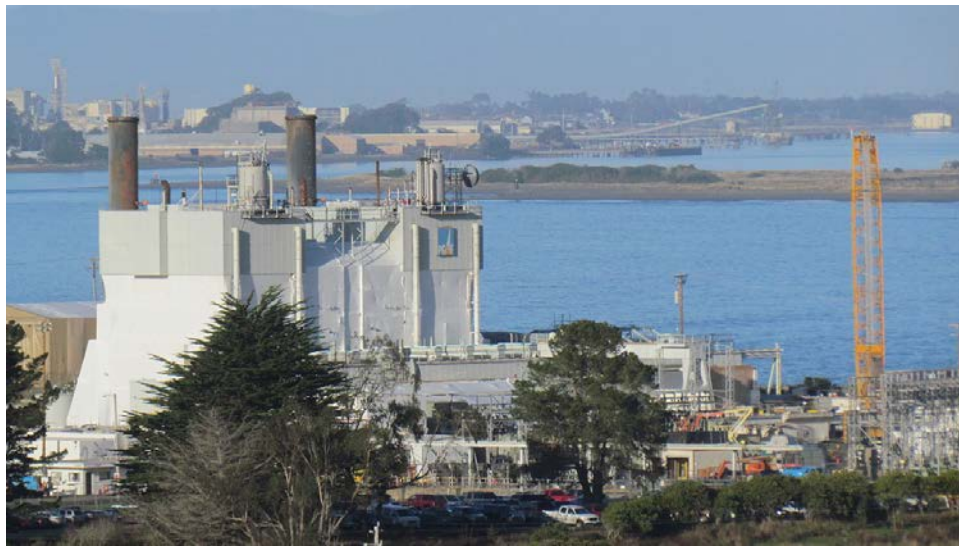
Figure 2: Humboldt Bay Nuclear Power Plant
