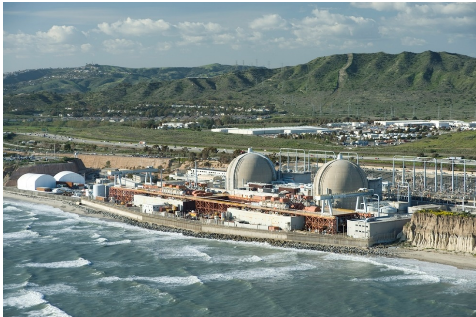
Figure 3: San Onofre Nuclear Generating Station
